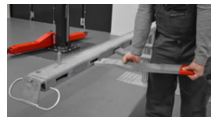
Fitting of lifting blades
